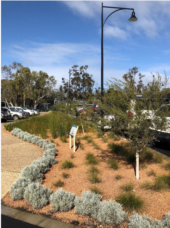
Figure 16. Example of a rain garden for stormwater quality management, at the City Administration building.
