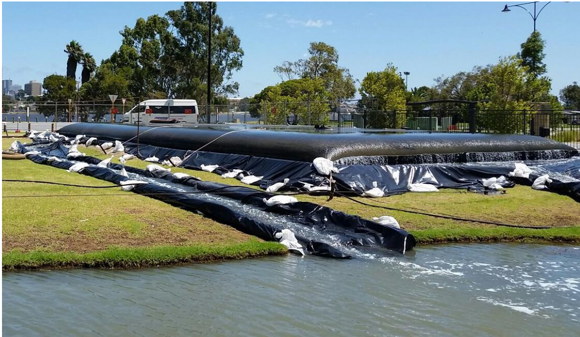
Figure 21. Geotextile bags used for sediment removal via dredging.
