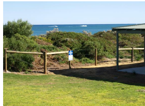
Treated pine post with ring-lock wire mesh ($30 - 40 per m 2 )
