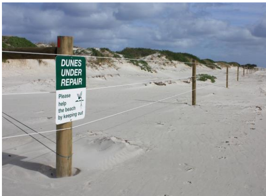
Treated pine post with PVC coated steel cable ($20 per m 2 )
