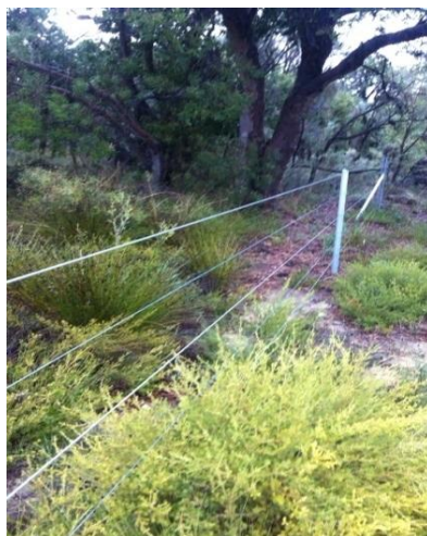
Heavy duty steel pole and steel cable fencing ($100 per m 2 )
