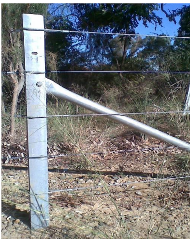
Heavy duty steel pole and steel cable fencing ($100 per m 2 )
